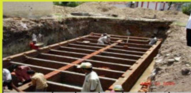
**Anaerobic Baffled Reactor**
